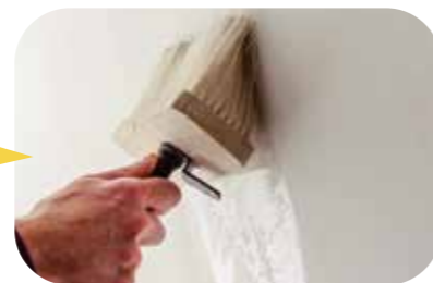
6. Apply a protective top coat and finish
