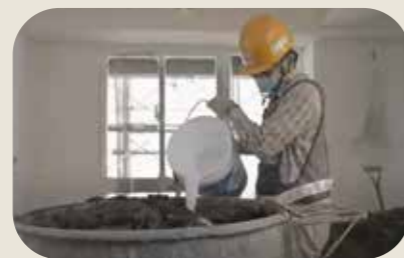
Add the diluted iwaterproof to the cement sand
