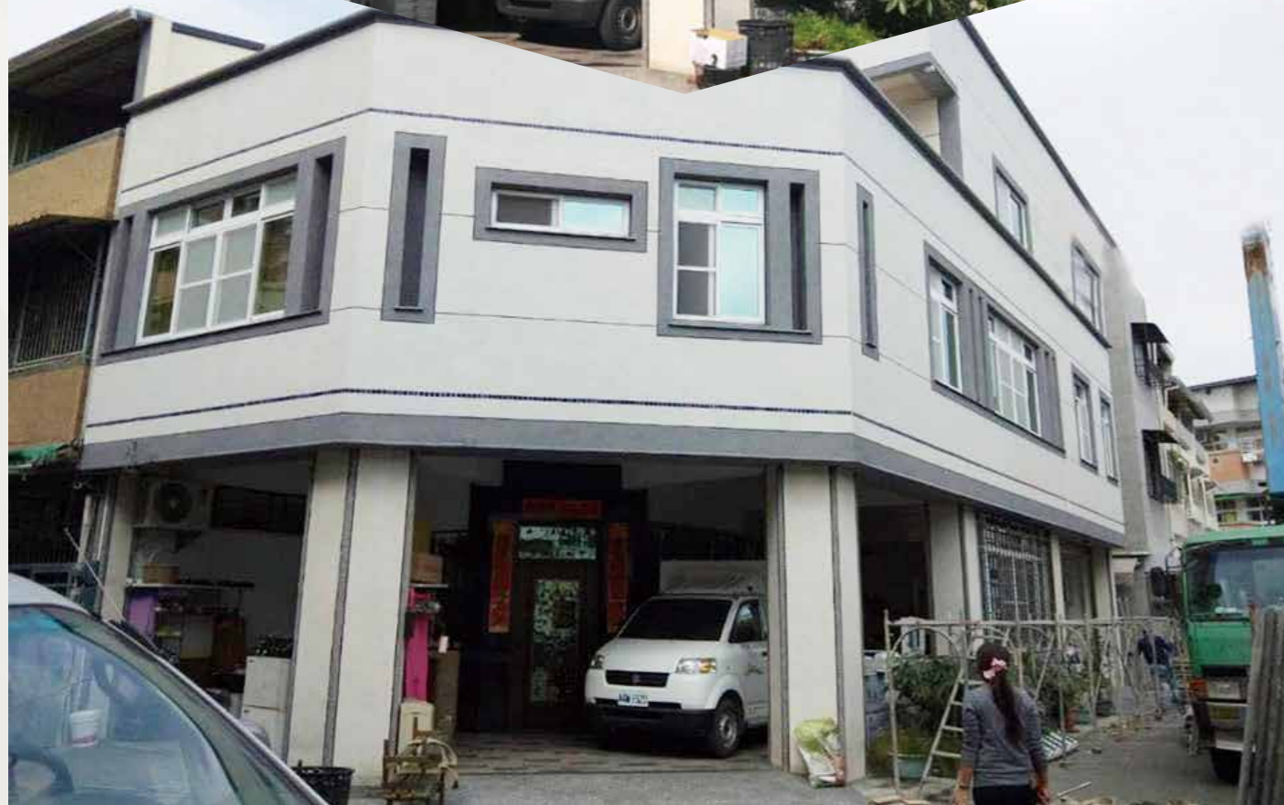
Private Home Renovation
